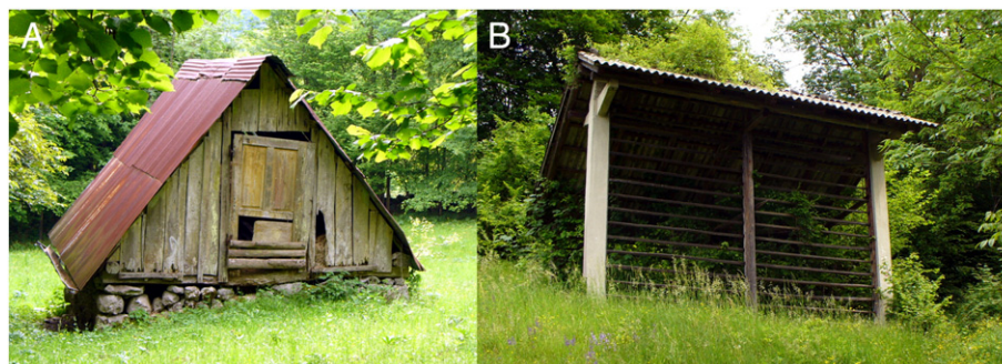
Fig. 3. Two examples of permanent scatterers. A) Example where the elevation change of -1.52 \text{ mm year}^{-1} is most likely associated with the decay of the shed. Because of this, it was not used in our study, despite the fact that it is in an area of active soil creep. B) Solid concrete foundations in a soil creep area on Carboniferous and Permian shales and sandstones. Such PSs were used for further data processing.
